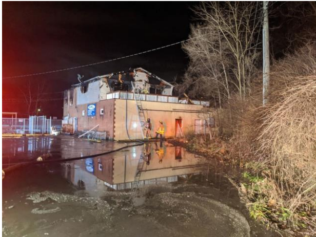
Valleyview Swim Club fire - J. Penty photo
